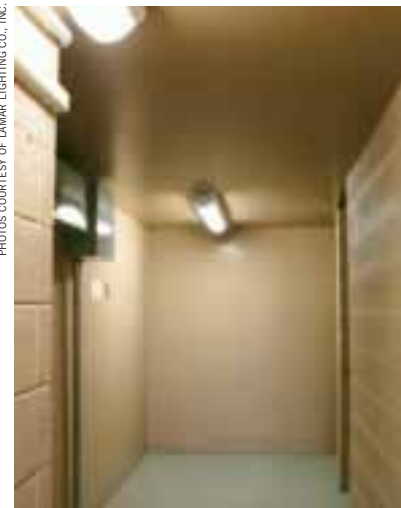
PHOTOS COURTESY OF LAMAR LIGHTING CO., INC.
